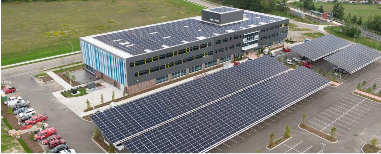
Figure 4. The evol1 green building in Waterloo, Ontario, Canada. Photo credit: The Cora Group.
